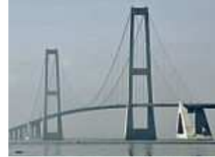
Great Belt Bridge
