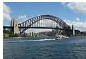
Sydney Harbour Bridge
