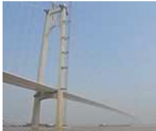
Nanjing Yangtze Bridge
