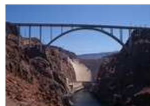
Mike Tillman Memorial Bridge
