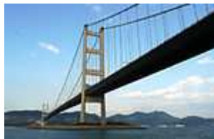
Tsing Ma Bridge
